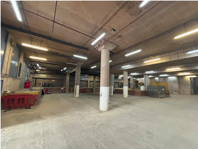
Fig 10 - Site Photo of Ground Floor Lvl/2
