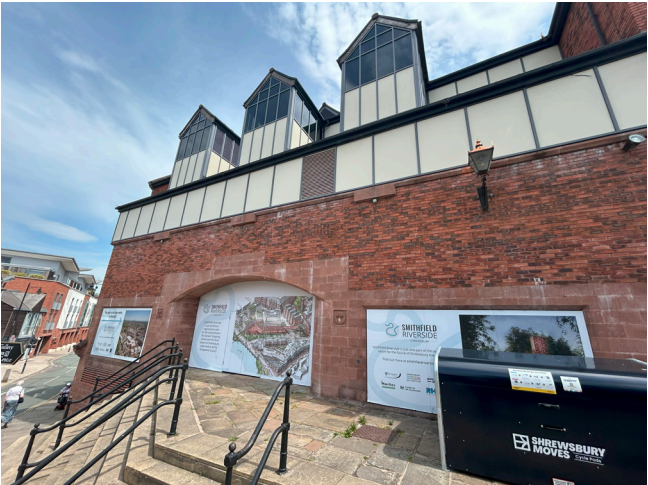
Fig 09 - Site Photo of Roushill Entrance
