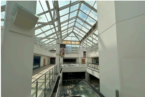
Fig 05 - Site Photo of Atrium
