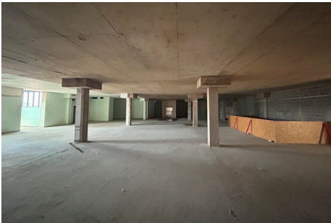
Fig 06 - Site Photo of Retail Unit
